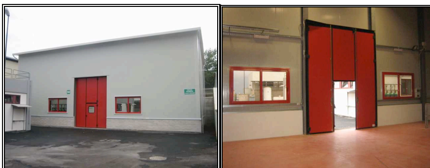
Figure 2: FLAME building at LNF completed on 23rd June 2008.
