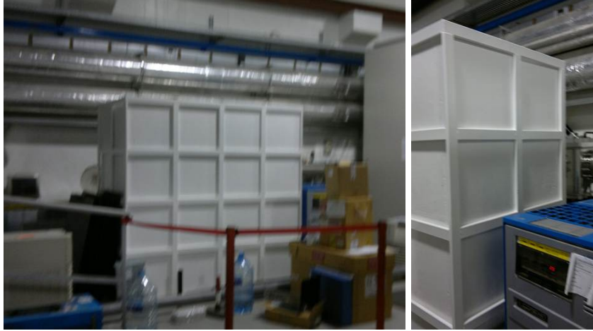
Figure 19: Concrete labirynth wall realized in front of the FLAME to SPARC bunker laser beam access, for shielding radiation (left). On the right a detail of the wall connection between the two experimental areas
